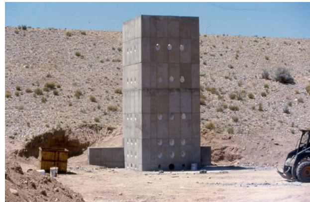
Figure 10. Completed Inclined Port Spillway Tower at South Baca Dam
