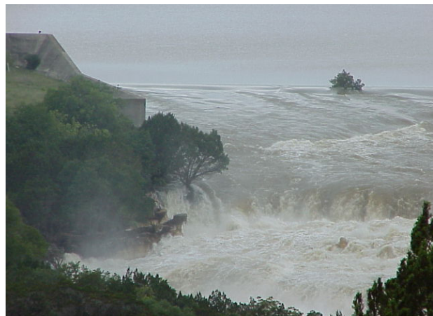
Figure 2. Canyon Lake Spillway Being Breached for the First Time Ever in the Early 90s
