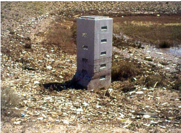
Figure 8. Trash Collector at Amole Dam
