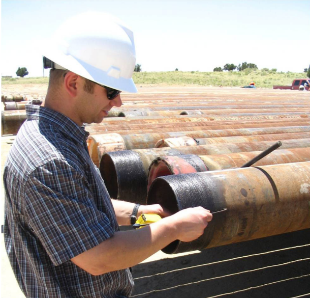
Figure 12. An On-Site OSE Inspector Measuring Casing Wall Thickness
