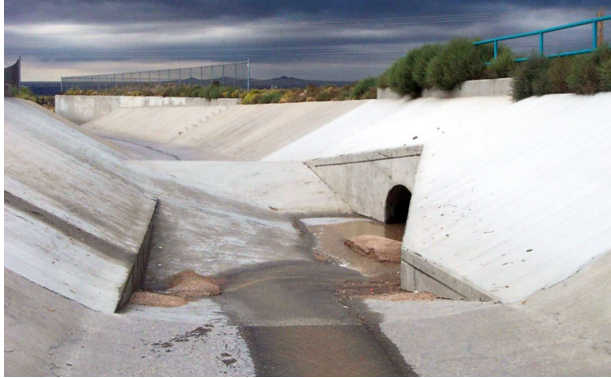
Figure 11. North Pino Channel Debris Intake Structure
