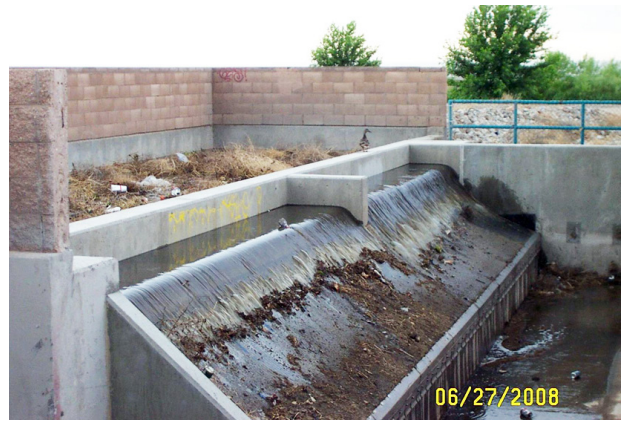
Figure 17. North Pino Coanda Screen Operation
