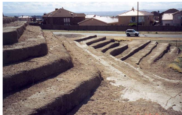
Figure 3. Kinney Dam Spillway
