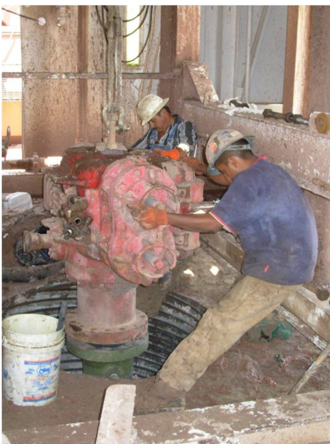
Figure 17. Attaching of the Blowout Preventer to the Casing
