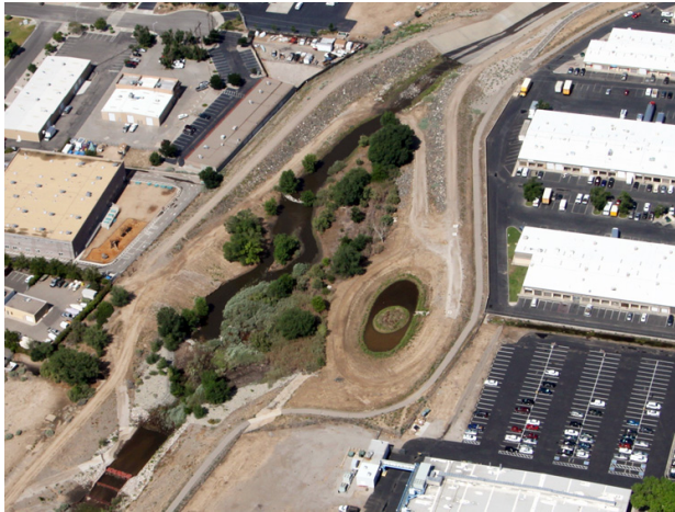
Figure 22. Bear Canyon Inlet Bio-Swales
