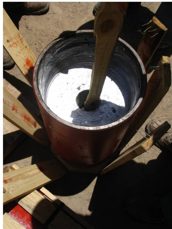
Figure 14. Cementing Shoe
