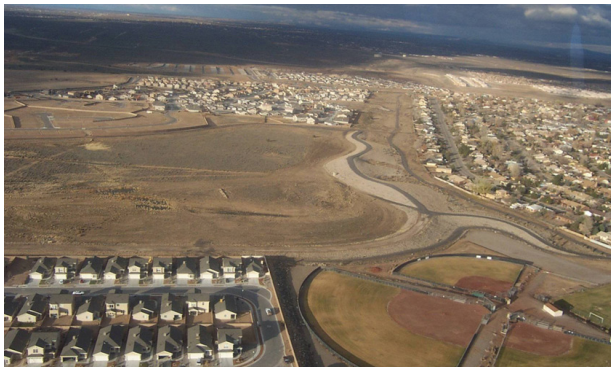
Figure 4. Las Ventanas Detention Dam
