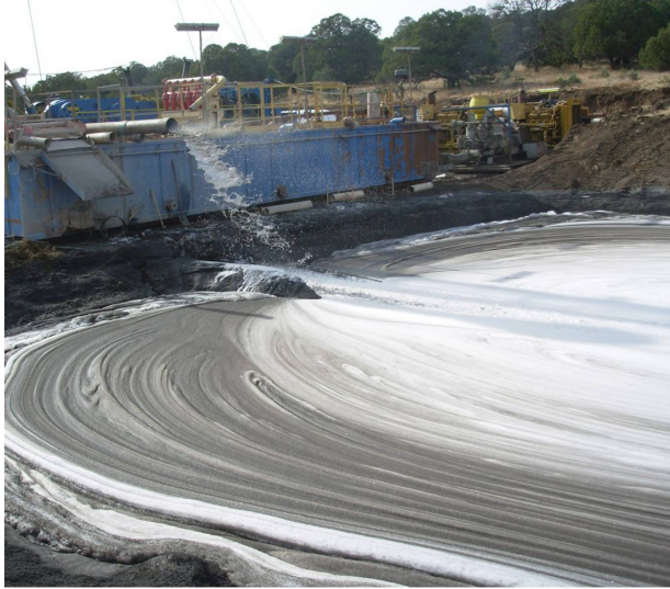
Figure 10. Hubbard Deep Well Initially Drilled on Air/Form
