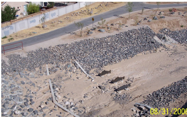
Figure 5. West I-40 Diversion Channel
