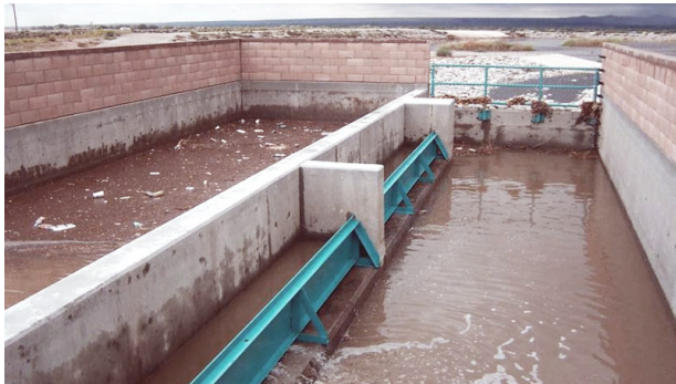
Figure 12. North Pino Arroyo Debris Removal Structure
