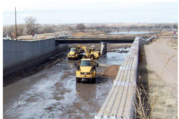
Figure 21. Sediment Removal at North Diversion Channel
